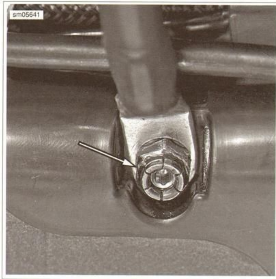
Figure 7-13. Negative Battery Cable Ground
