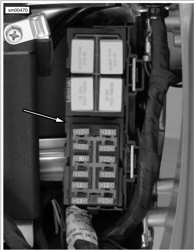
Figure 6-76. Fuse Block and Main Fuse Location: Ulysses
