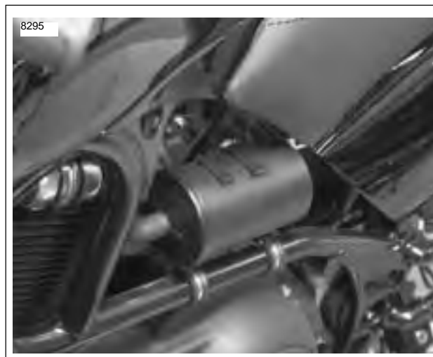
Figure 4-110. Carbon Canister Installation (Typical).
