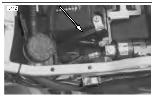
Figure 7-36. Negative Battery Cable
