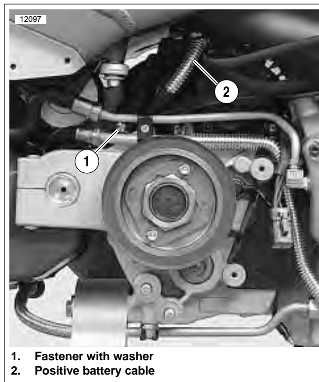
Figure 7-40. Positive Battery Cable (Protective Boot Not Shown)
