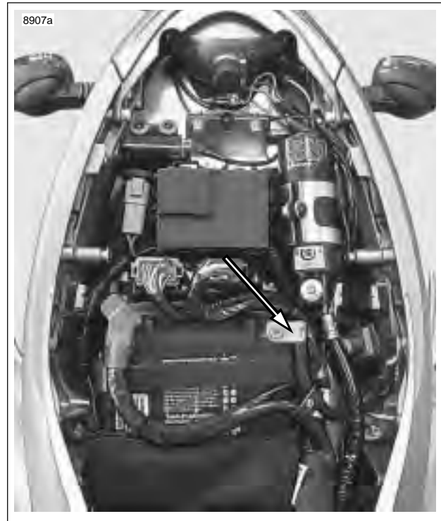
Figure 7-44. Negative Battery Cable
